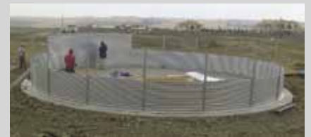
Completion of the first ring
