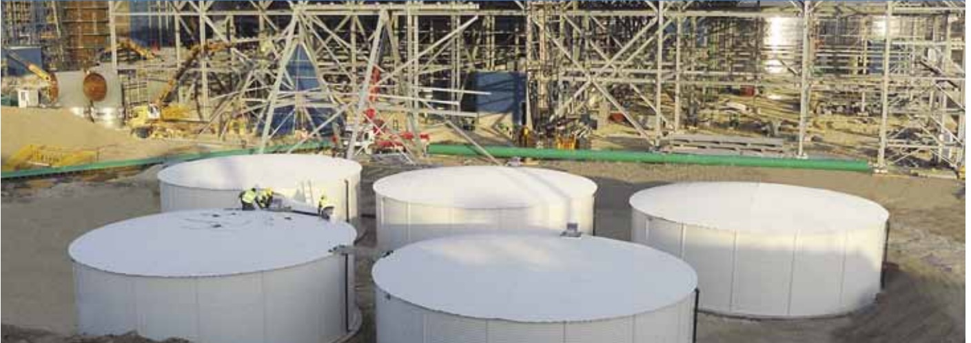
Dilovasi, Gebze - Izmit / Turkey 865MW Natural Gas Power Plant Project, 5 Demi Water Storage Tanks with 255 m 3 Capacity, Apollo Type
