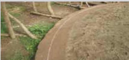
Marking out the tank diameter
