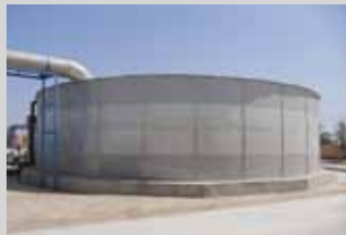
Industrial water supply
