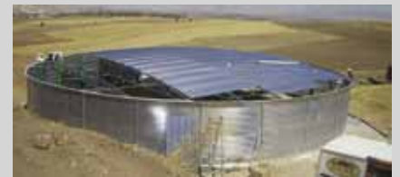
Laying and fitting on the roof sheets across the truss
