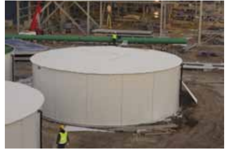
Dilovasi, Gebze - Izmit / Turkey 865MW Natural Gas Power Plant Project, 5 Demi Water Storage Tanks with 255 m 3 Capacity, Apollo Type
