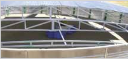
Completion of the roof top
