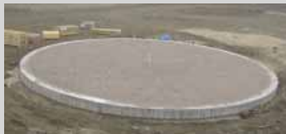
Checking out the concrete ring foundation and sand pad
