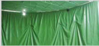
Fitting and securing the flexible liners
