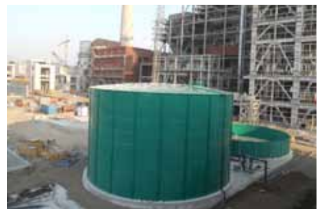
Aliaga - Izmir / Turkey 488MW Natural Gas Power Plant Project, 2 Demi Water Storage Tanks with 1.433 m 3 Capacity, Apollo Type
