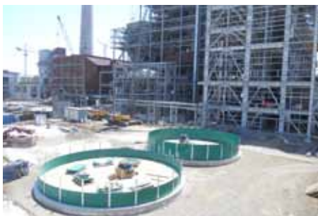
Aliaga - Izmir / Turkey 488MW Natural Gas Power Plant Project, 2 Demi Water Storage Tanks with 1.433 m 3 Capacity, Apollo Type
