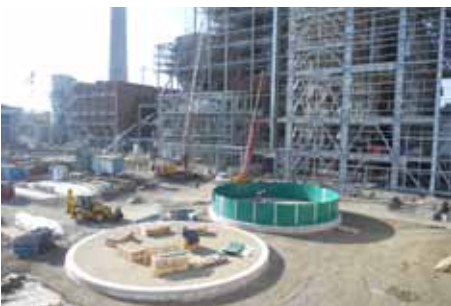
Aliaga - Izmir / Turkey 488MW Natural Gas Power Plant Project, 2 Demi Water Storage Tanks with 1.433 m 3 Capacity, Apollo Type
