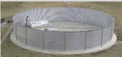
Installation of the remaining panels
