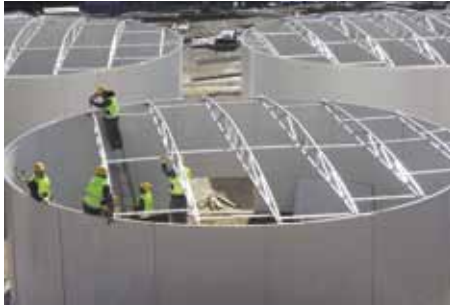
Dilovasi, Gebze - Izmit / Turkey 865MW Natural Gas Power Plant Project, 5 Demi Water Storage Tanks with 255 m 3 Capacity, Apollo Type
